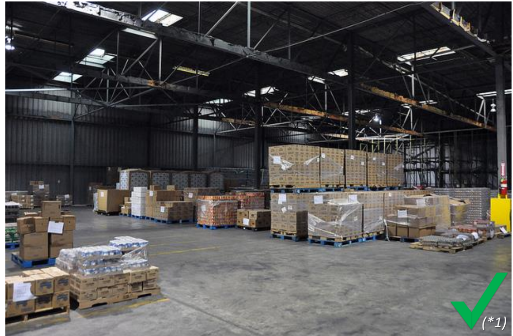
Warehouse with good housekeeping and a designated aisle way.
