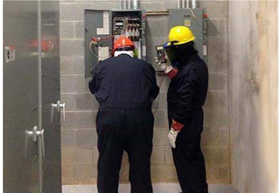
Electrical workers using proper personal protective equipment. (*7)
